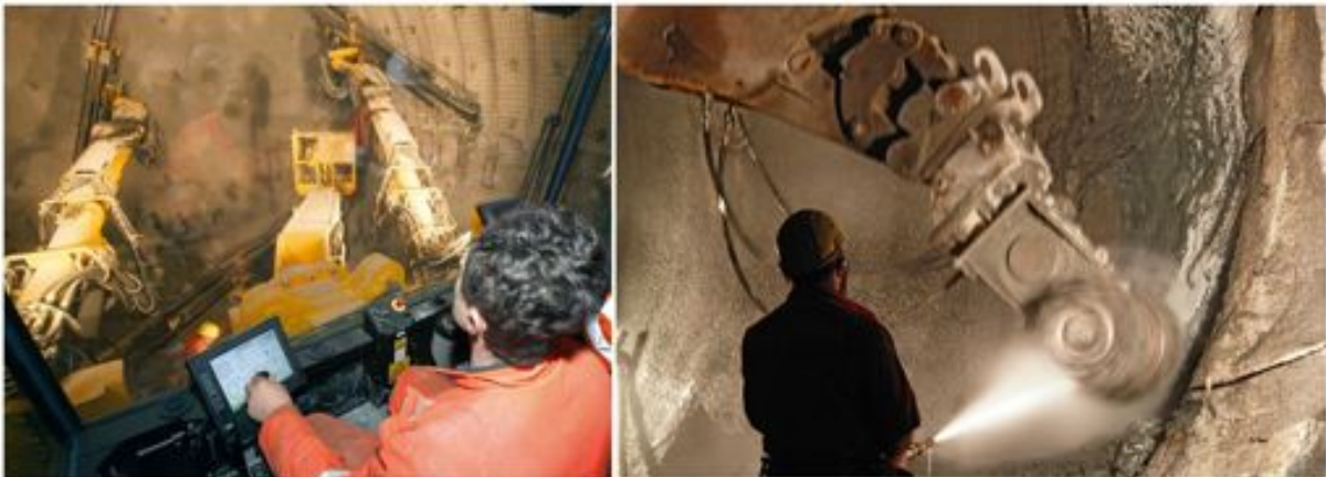
Figure 80: Special tooling has been developed for the D&B technique for tunneling.
