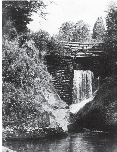
Fig. 7 – The stua of Ramàz at the end of its opening (from Fabbroni Grillo 1977)
