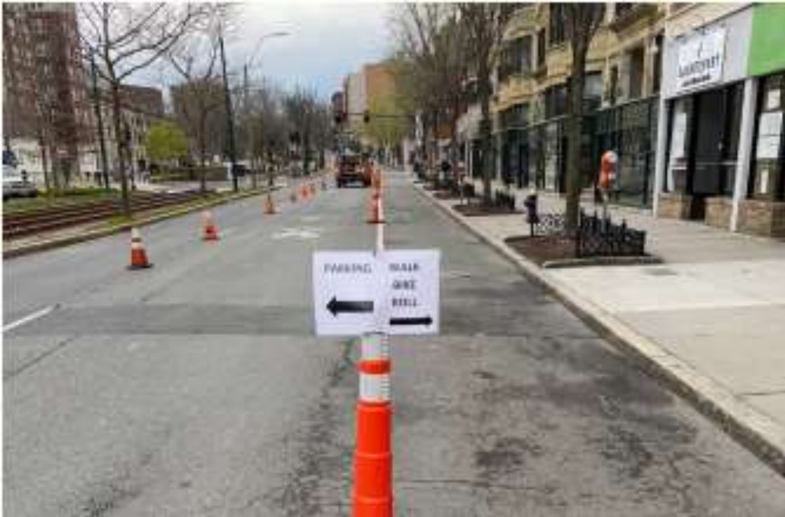
Fig.7 Brookline (MA, USA) used cones and temporary signs mounted on freestanding delineator posts to extend sidewalks and create bike lanes along four high-volume streets (Source: https://nacto.org/wp-content/uploads/2020/07/200708_Sidewalk-Extensions.pdf )
