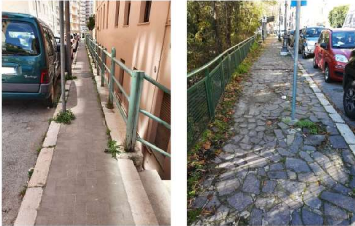
Fig.3 A frequent sidewalk type with bidirectional flow in non-renewal residential area of Potenza, a medium-size regional capital of a City of South Italy region, infrastructure characterized by a width just enough the walking of just one person
