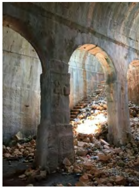
Fig. 6 – Inner view of the Cistern
