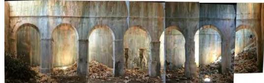
Fig.9-Longitudinal view of the arches in the Cistern
