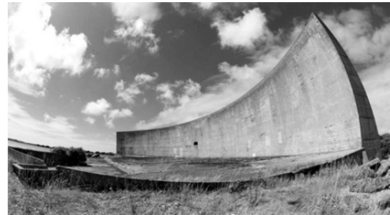
Figure 6. Top: Some aerophones from France and Italy, Bottom: Sound mirror - 60 meters long – in Dengie, Great Britain. In the area of concrete in front of the wall the researcher William Sansome Tucker installed 20 microphones for a better search for the direction of arrival of the aircraft.
