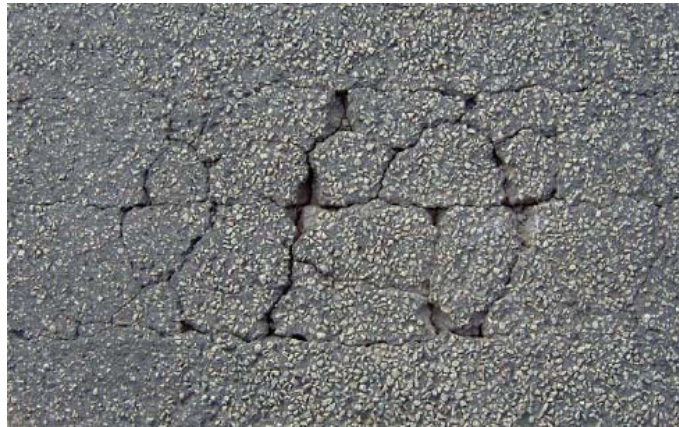
FIGURE 2-20 Visual observations indicating deck plate crack (Dong et al., 2004)
