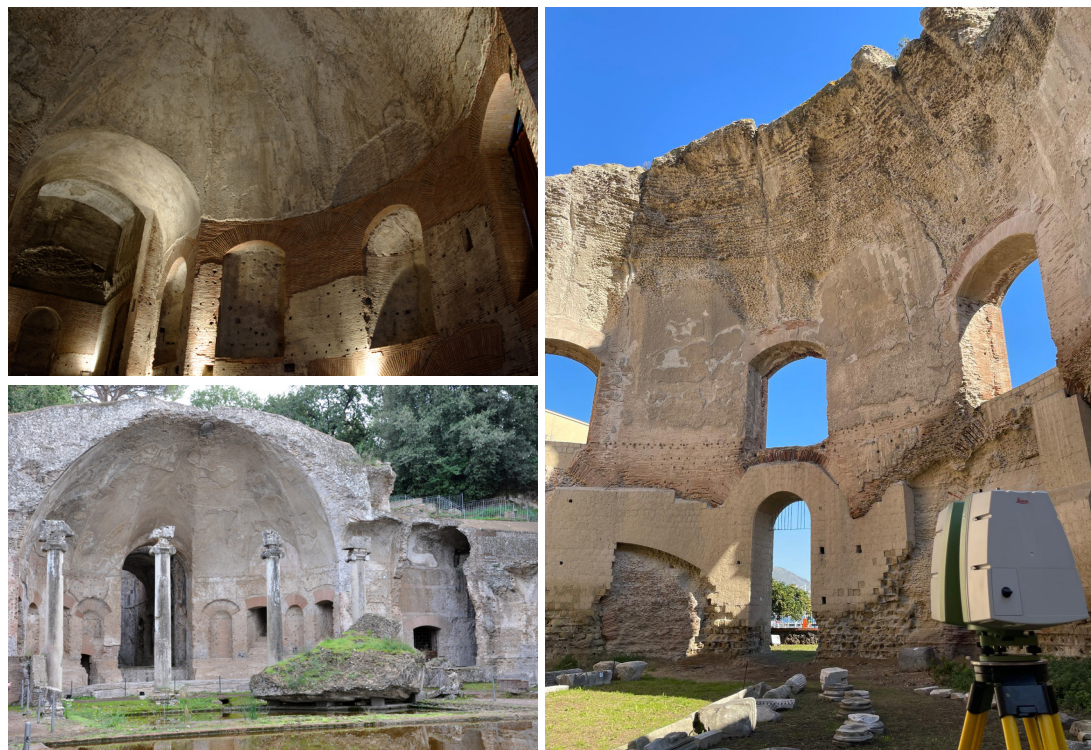
Fig. 1 - Segmental Hadrianic vaults on circular layouts: (top) Horti Sallustiani, Rome; (bottom) Serapeum, Hadrian's Villa, Tivoli; (right) Temple of Venus, Baiae, Bacoli.
