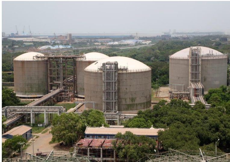
(Figure.14. Double Integrity Cup Storage Tank)
