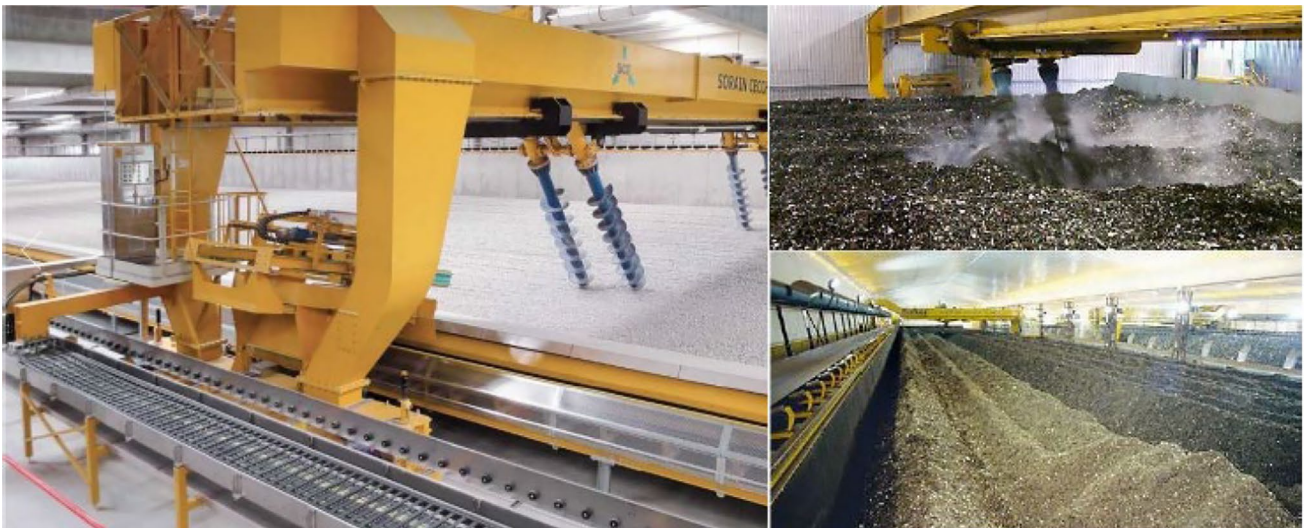
Fig. 2 Aerobic bioreactors in the studied MBT plant
