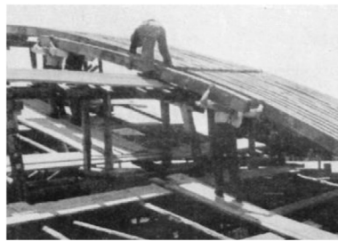
RDB, S.A.P reinforced brick vault, 1939 (Bari)
