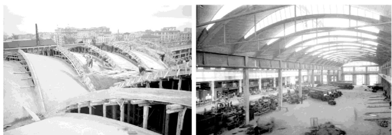
Figure 2. Cast in-place reinforced concrete thin shells: a) iron manufacturing department of the Cantieri Riuniti dell'Adriatico (CRDA) in Panzano (Monfalcone), b) warehouse of CRDA in Panzano, c) tracing building for the Ansaldo shipyards in Genoa, d) tower assembly workshop for the Ansaldo shipyards in Genoa, e) warehouse for the hemp in Tresigallo (Ferrara), f) ATAG Central Workshops in Rome
