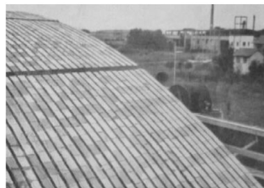
RDB, S.A.P reinforced brick vault, 1939 (Monza)
