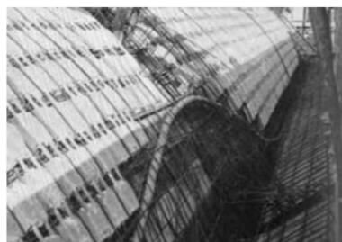
Figure 3. Semi-prefabricated thin vaults in reinforced brick: a) S.A. Cementi plant in Monopoli (Bari), b) ponificio Ambrogio Silva in Seregno (Monza), c) prototype of a thin vault in reinforced brick by Giulio Pizzetti, d) large hall of the Officine Biraghi mechanical workshop in Milan
