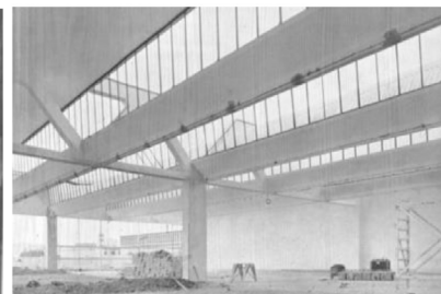
Figure 3. Semi-prefabricated thin vaults in reinforced brick: a) S.A. Cementi plant in Monopoli (Bari), b) ponificio Ambrogio Silva in Seregno (Monza), c) prototype of a thin vault in reinforced brick by Giulio Pizzetti, d) large hall of the Officine Biraghi mechanical workshop in Milan
