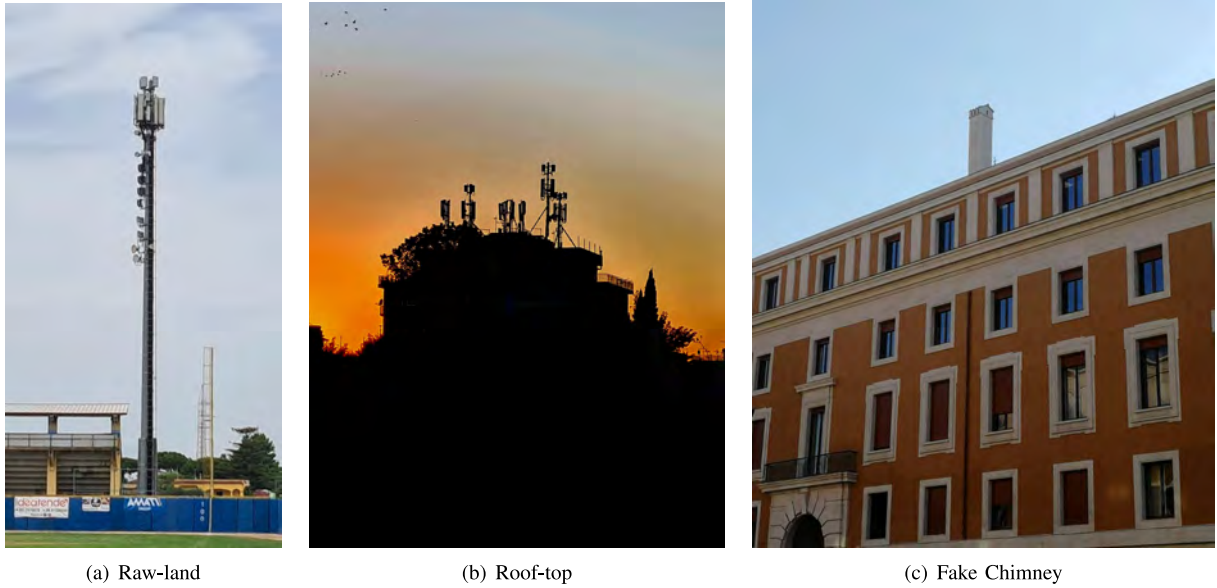
FIGURE 4. Main types of cellular towers.
