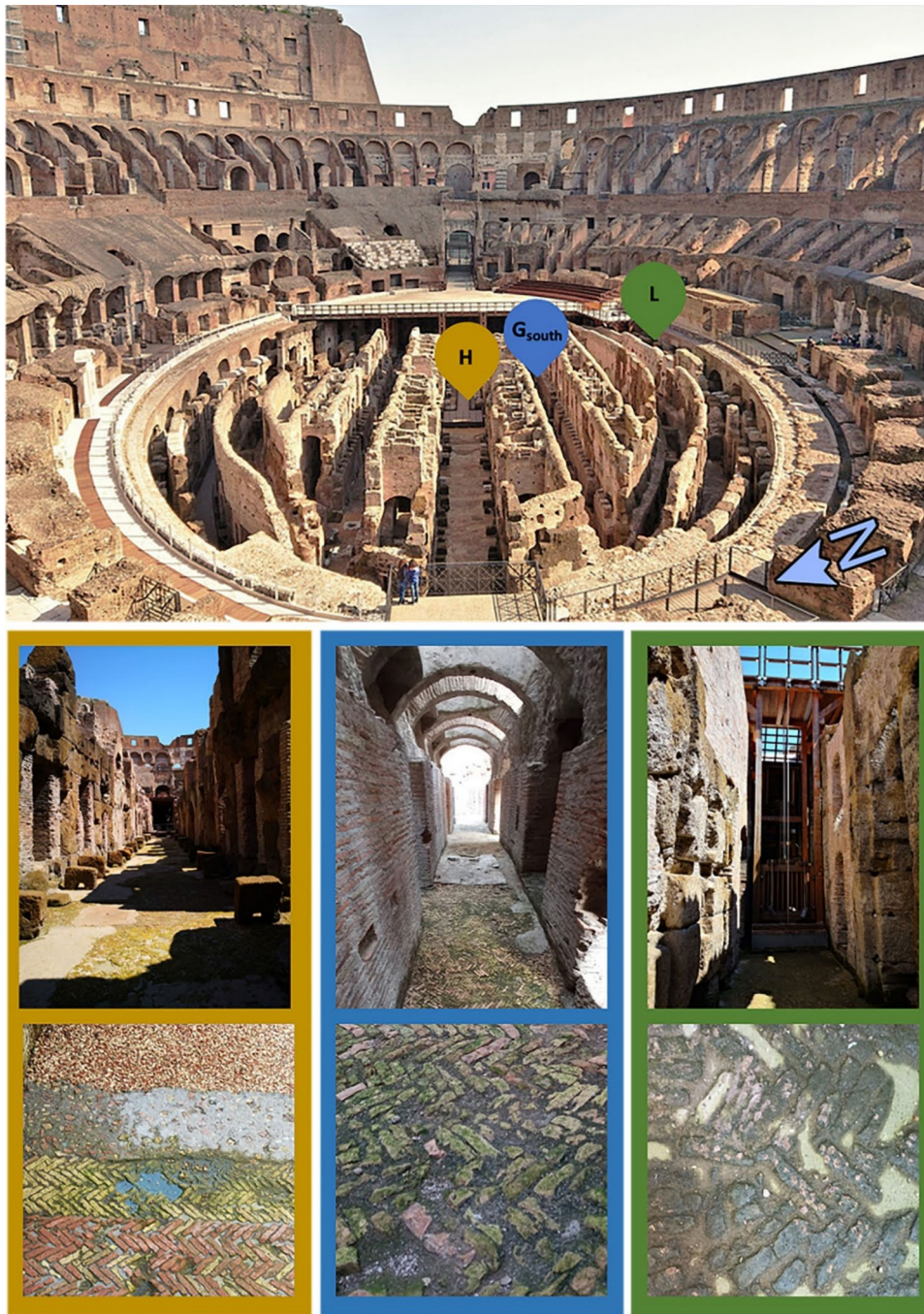
Fig. 1 Selected areas in the Colosseum hypogeum: H (in yellow), G-south (in blue) and L (in green) sites are characterized by different environmental conditions and different construction materials and techniques, “cocciopesto” and “ opus spicatum ” floors
