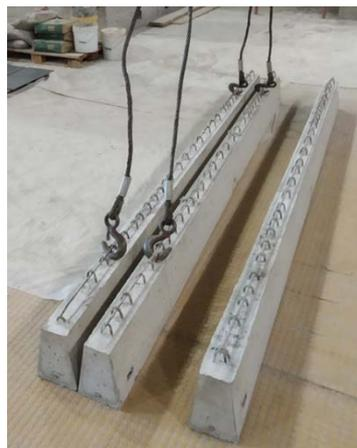
Figura 5.20: Travi prefabbricate in c.a.p..
