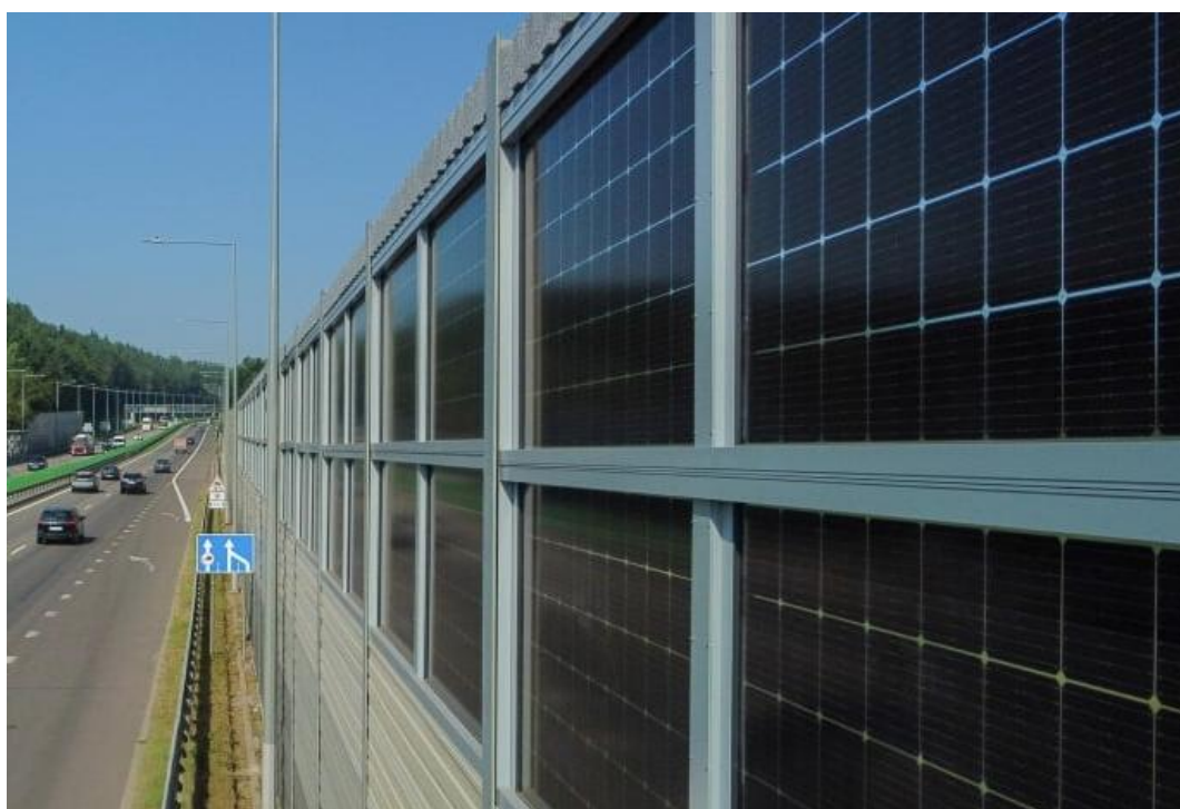
Figure 14 – Photovoltaic noise barriers in Lithuania [115].
