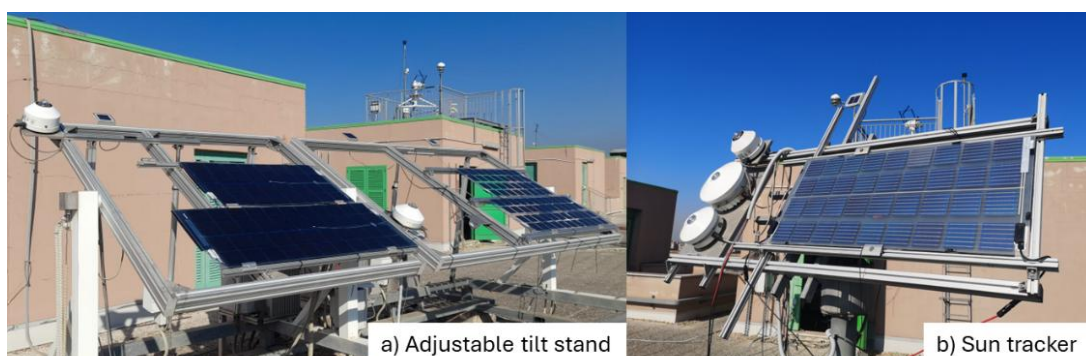
Figure 15 – Equipment used for the execution of the procedure
