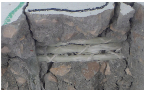
Fig. 10. Bending test results of CSA/GFRP (I) segment (26 hours aged): detail of the tensile failure of the GFRP bars (at mid-span of the intrados surface).
