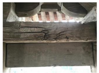
Figure 3. Damaged beam with knots
