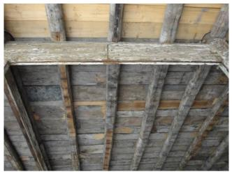
Figure 1. Cracks in square beam
