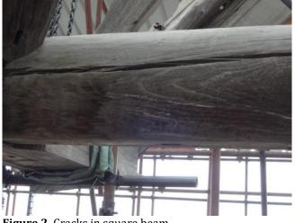
Figure 2. Cracks in square beam
