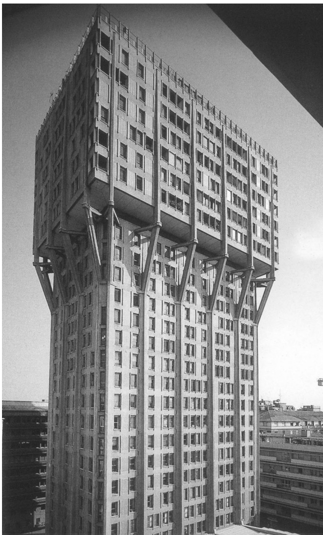
Figure 1. Velasca tower, Milan. General view.
