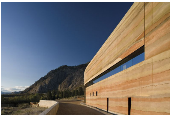
Fig. 9: Muro in pisè, Nk'mip Desert Cultural Centre, Canada, 2008
