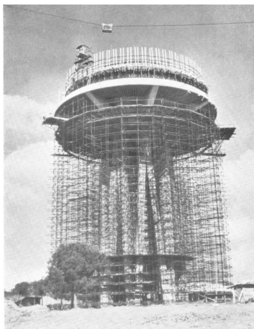
Figure 6. Roberto Colosimo Sr with Aldo Capozza and Sergio Varisco, view of the EUR Water Tower, Rome, 1957-59 the construction site was served by two antennas and a blondin .
