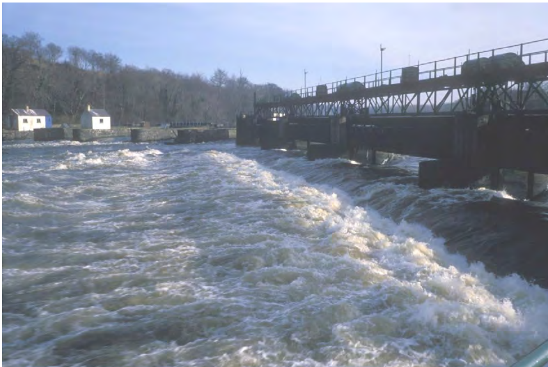
Figure 3.2. Sluice gates on the Bann corridor.
