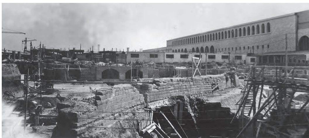
Fig. 7 The internal retaining wall of the Esquilinus agger : rescue excavations at Stazione Termini, 1948 (after Cifani 2008).
