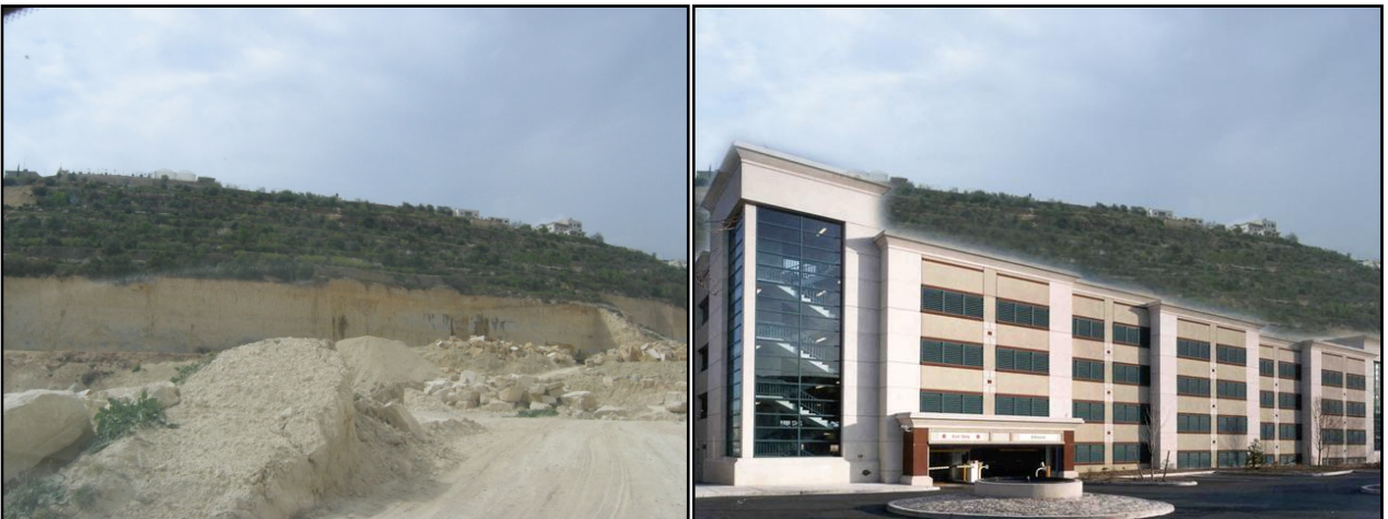
Figure 7.10: Current view and a future possible view (not to scale) for Quarry number 73 (Injas Area designated rehabilitation Plan) which is supposed to be rehabilitated as a commercial center .
